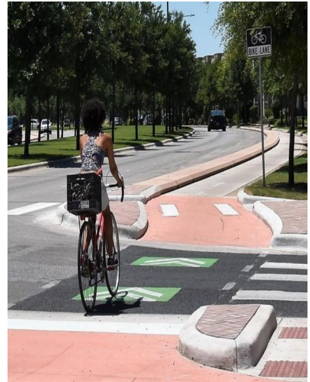
arated bike lane using a concrete curb in Austin, TX, USA that considers context in selection of facility type. Source: City of Au.
