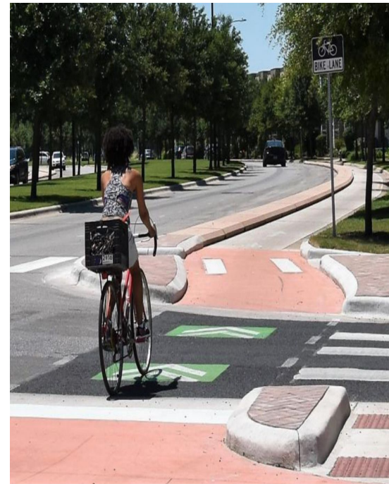
ated bike lane using a concrete curb in Austin, TX, USA that considers context in selection of facility type. Source: City of Au.
