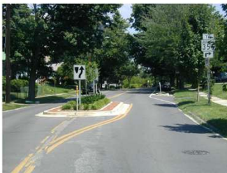
Figure 8-5: Example of a Chicane Treatment on a Two-Way Street Created by a Median and Curb Extensions
