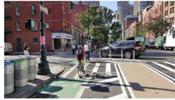
Figure 7-15: Corner Island with Flexible Delineator Posts (Source: Carl Sandstrom, PE, Office of Bicycle and Pedestrian Programs, New York City Department of Transportation)
