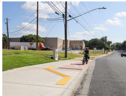
Detail 1—Preferred bicycle ramp alignment with wide sidewalk buffer
