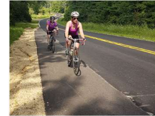
Figure 12-3: Shoulder Widening on Uphill Section of Roadway to Accommodate Bicycling
