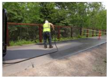
Figure 15-4. Pop Sealing a Shared Use Path
