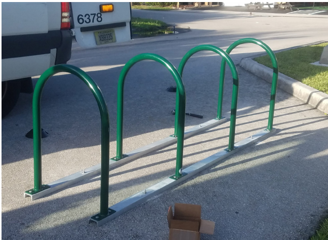
Installation of bike racks on asphalt surface in Fort Lauderdale, FL. (Photo credit: Mauricio Hernandez)
