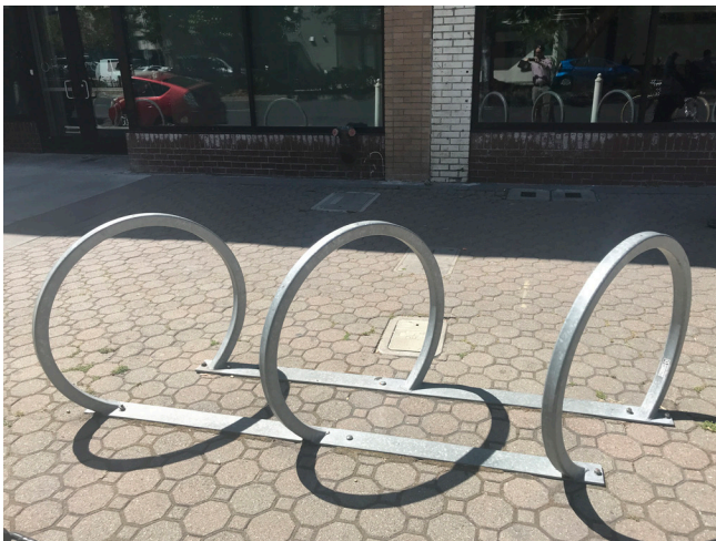
Welded steel flat bar rail-mounted racks anchored to concrete pavers, Oakland CA (Photo: Heath Maddox)
