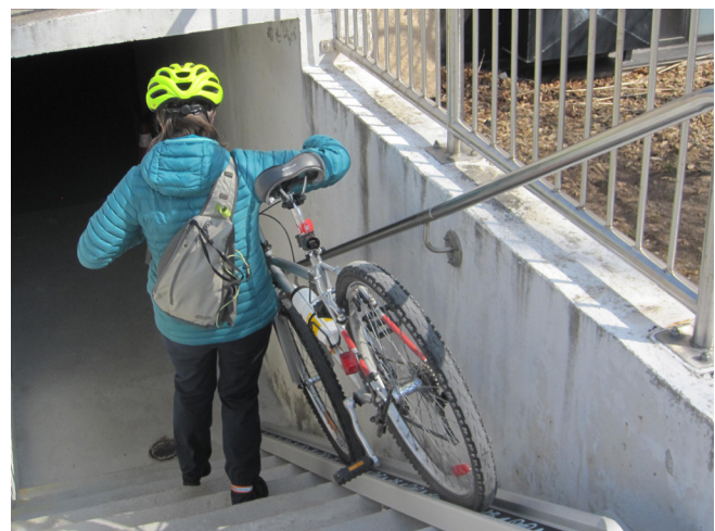
Bike stair ramp to access parking garage bike lock-up in London, Ontario (Photo: Allison Miller)
