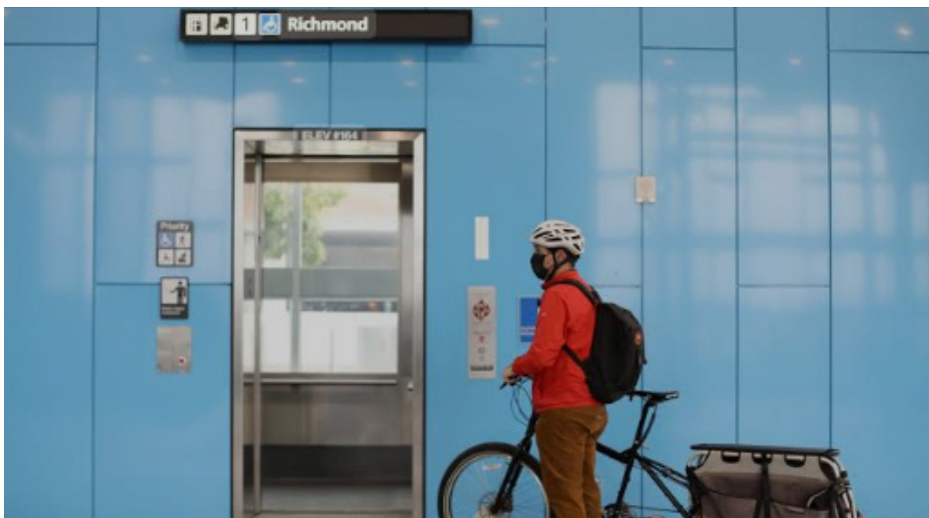
Accessible elevator for cargo bikes at El Cerrito del Norte BART Station. El Cerrito, CA (Photo: Heath Maddox)
